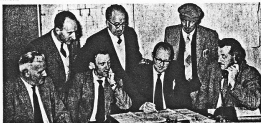
In the site office. Standing l. to r.: D. Dwane, F'man Carpenter; J. Jennings, Timekeeper/checker; S. Sharpe, Finishing F'man; Seated l. to r.: W. Morrison, S'keeper; K. Pryor, F'man Carpenter; R. Horne, Gen. F'man and M. Griffin, Gen. F'man in charge
